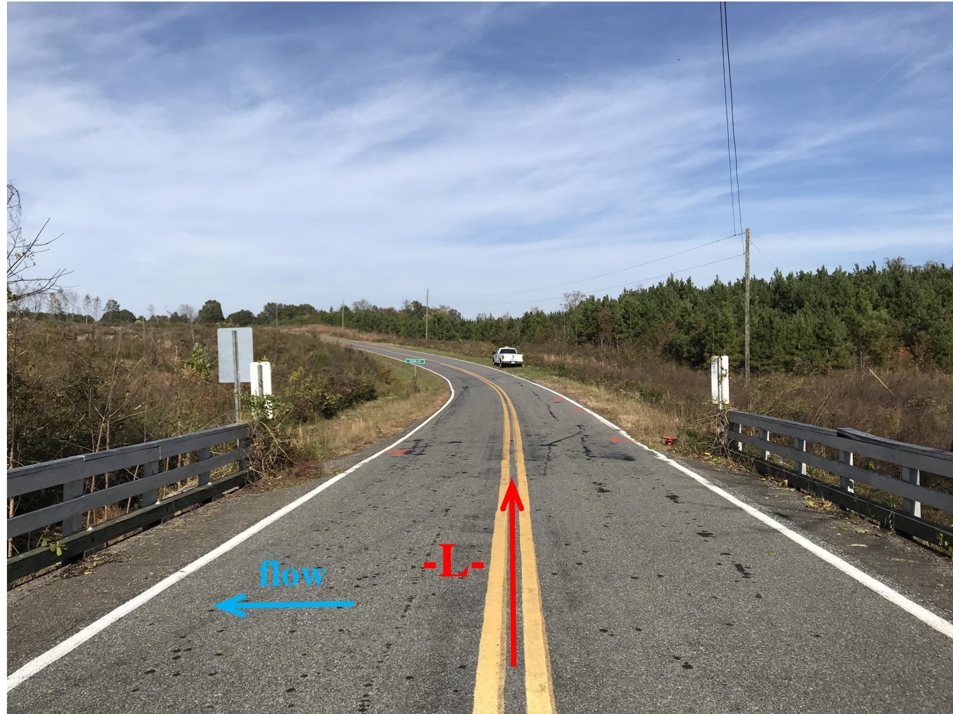
Looking Upstation toward Marys Grove Rd
